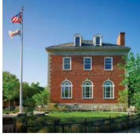
Northeast Neighborhood Library
